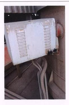
**CEMS installed for Cement Mill**
